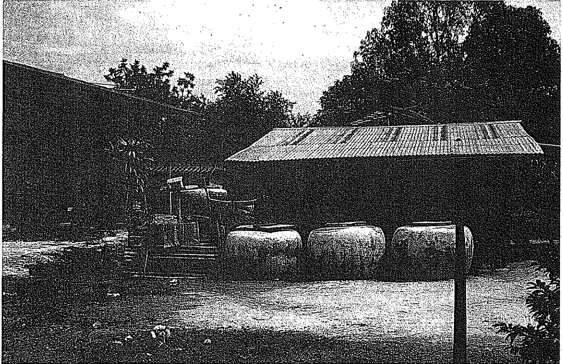
Figure 3.15: Rainwater harvesting from rooftops in northeastern part
